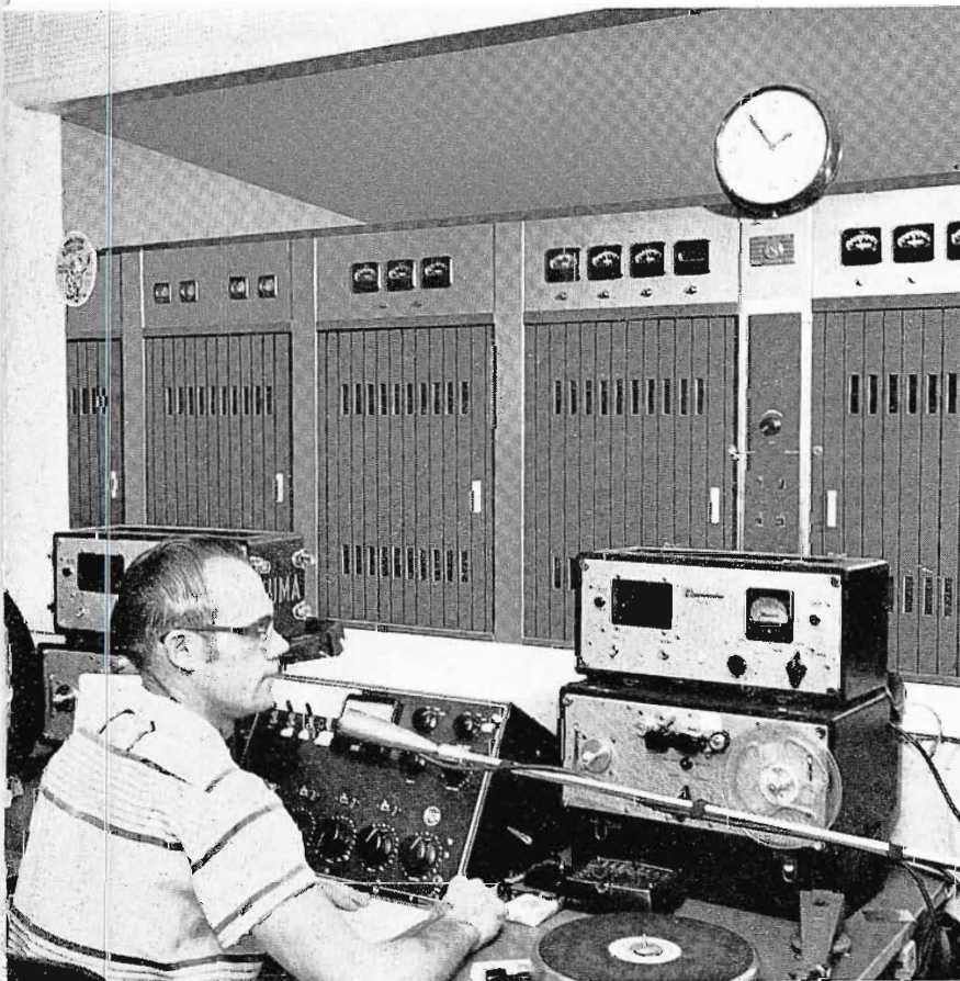
FIG. 25. Transmitter control location includes all facilities for program origination. Here a BC-5A consolette handles all program requirements.
