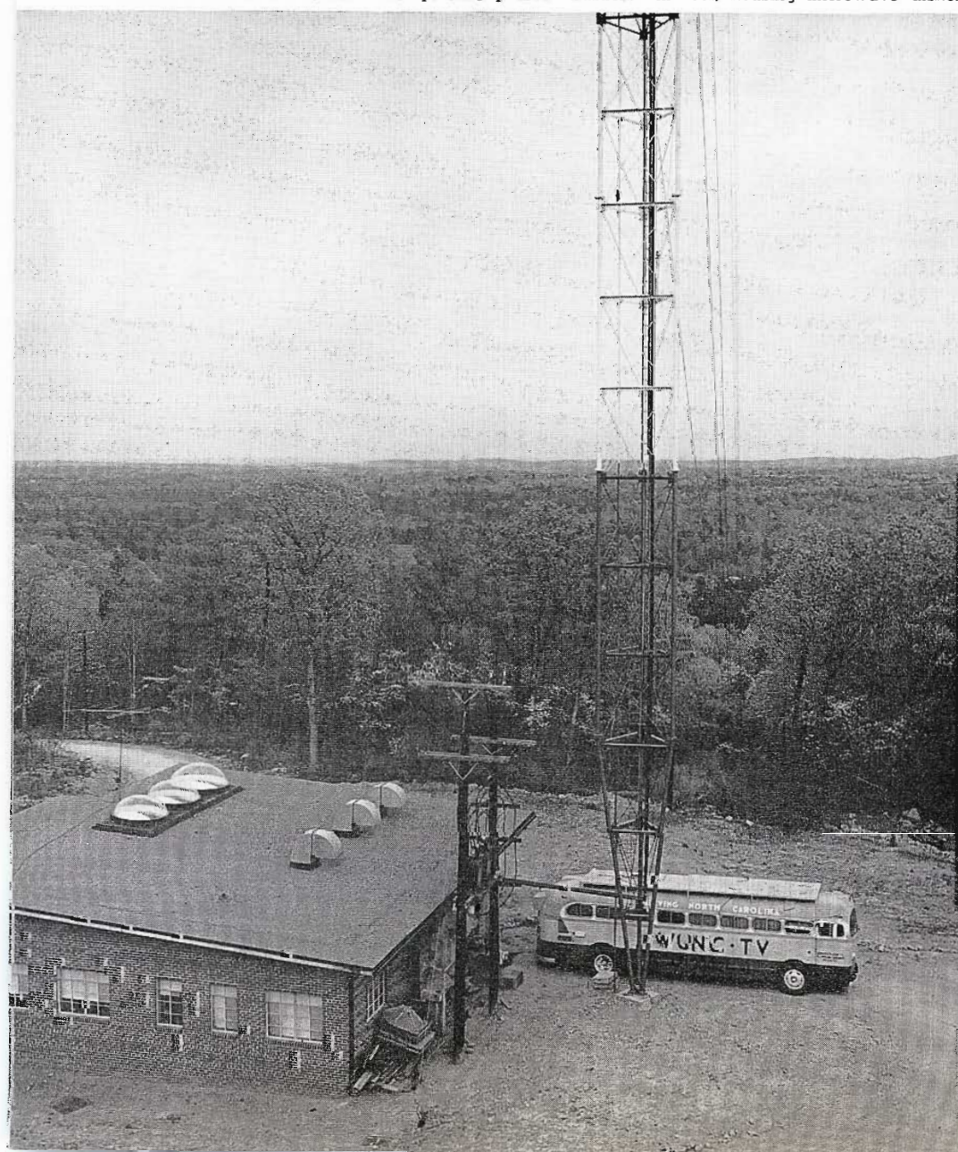
FIG. 36. WUNC-TV transmitter site is approximately eight miles southwest of Chapel Hill, atop Terrell's Mountain, Chatham County. Note plastic "bubbles" in roof, housing microwave dishes.
